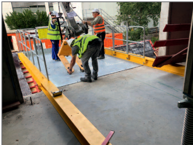
The aluminium props are simply folded up and fixed work platform is clearly visible
